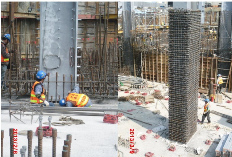
Figure 1 Steel Column Construction
