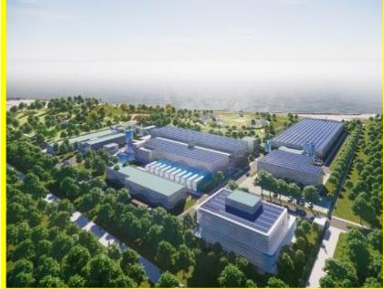
Hsinchu Desalination Plant
