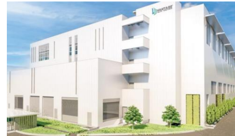
U.S. Company's Data Center (Taoyuan, Taiwan)
