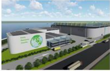
Low Carbon Recycling and Disposal Center (Changbin)
