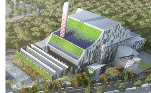
Biomass Energy Center (Taoyuan)
