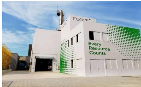
Waste Solvent Recycling Plant (Taoyuan)
