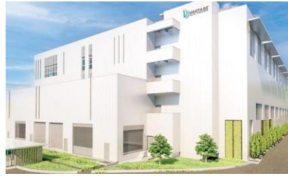
U.S. Data Center Building Project in Taoyuan, Taiwan
