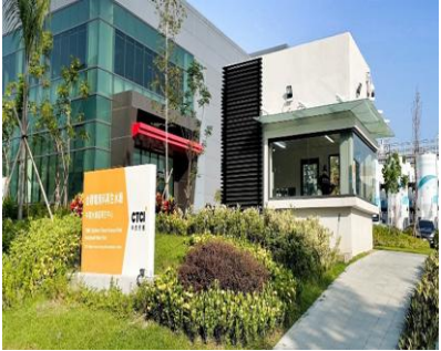
TSMC Tainan Science Park Reclaimed Water Plant
