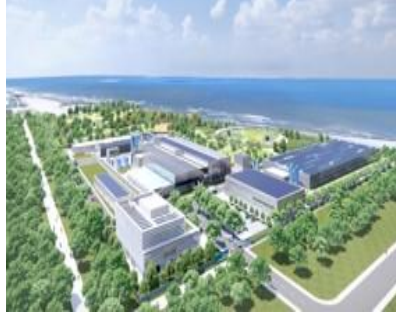
Hsinchu Desalination Plant Construction and Operation Maintenance
