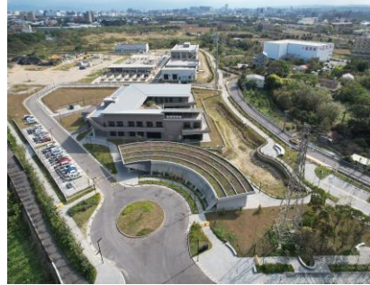
Construction of sewage sewer system in Zhongli area
