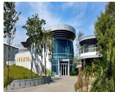
Kaohsiung Fengshan Creek Reclaimed Water Plant
