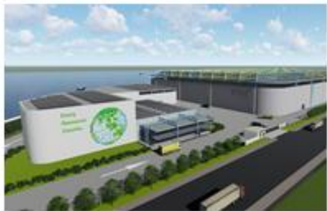
Low Carbon Recycling and Disposal Center (Changbin)
