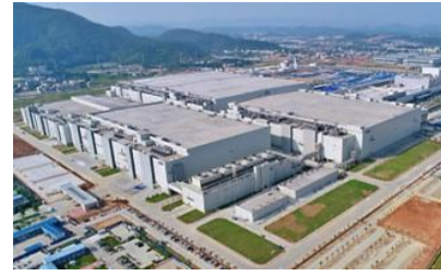
Guangzhou TFT-LCD Panel Plant Cleanroom Construction Project
