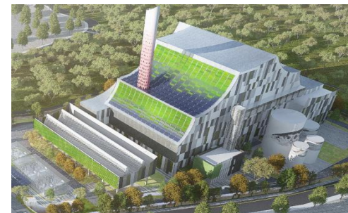
Biomass Energy Center (Taoyuan)
