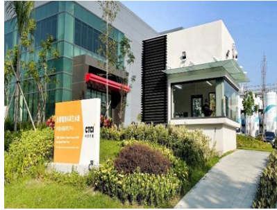
TSMC Tainan Science Park Reclaimed Water Plant
