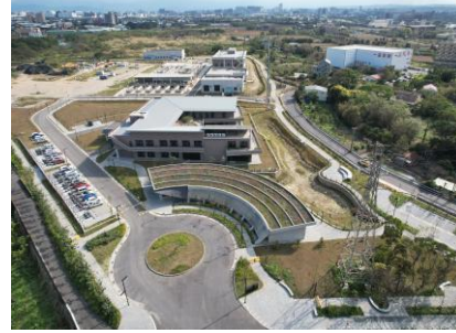
Construction of sewage sewer system in Zhongli area
