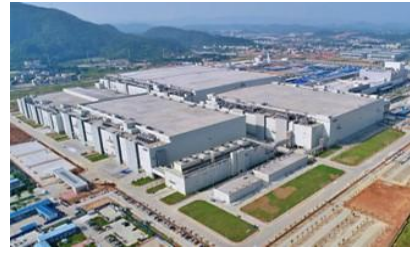
Guangzhou TFT-LCD Panel Plant Cleanroom Construction Project
