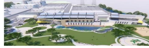
Kaohsiung Linhai Sewage Treatment Plant and Reclaimed Water
