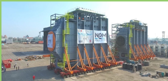
Modular construction applications
